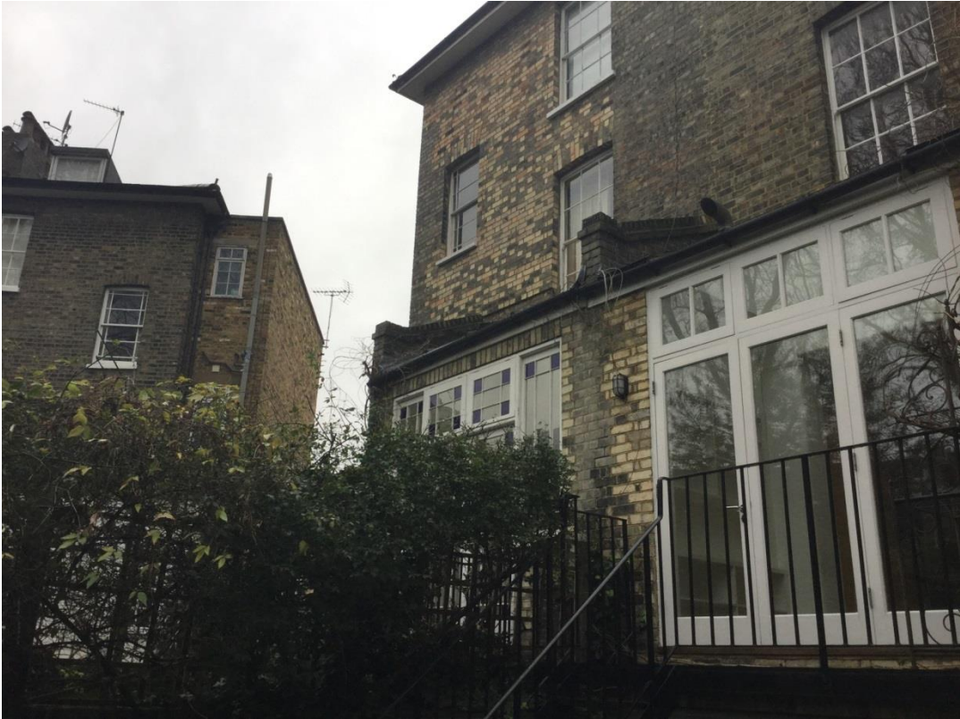
Image 2. The rear elevation of the site and No.29 Richmond Crescent.
